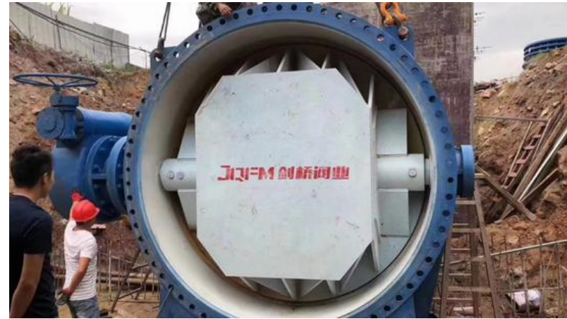
Installation DN3000 butterfly valve
